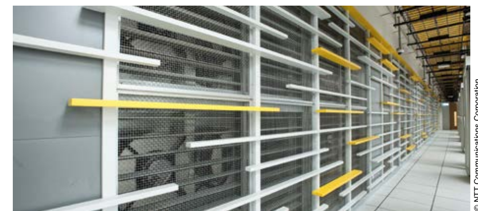
Front flow air handling unit in front of the server aisles
