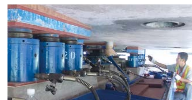
16 jacks beneath the bridge controlled by jack synchronous system
